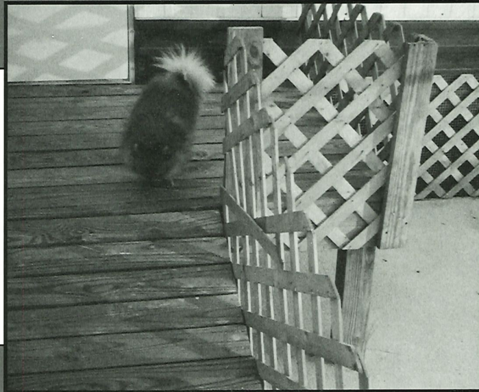
A ramp is constructed for the dogs from the kennel building. The land is flat so the ramps - along with the gravel - help with building strong legs. Sides were constructed for safety
